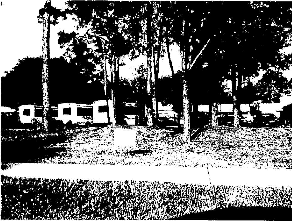
View of existing facility
